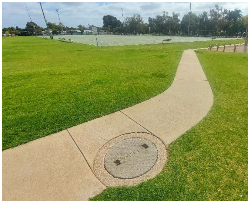
Figure 12 Existing concrete pavement looking north towards netball courts
