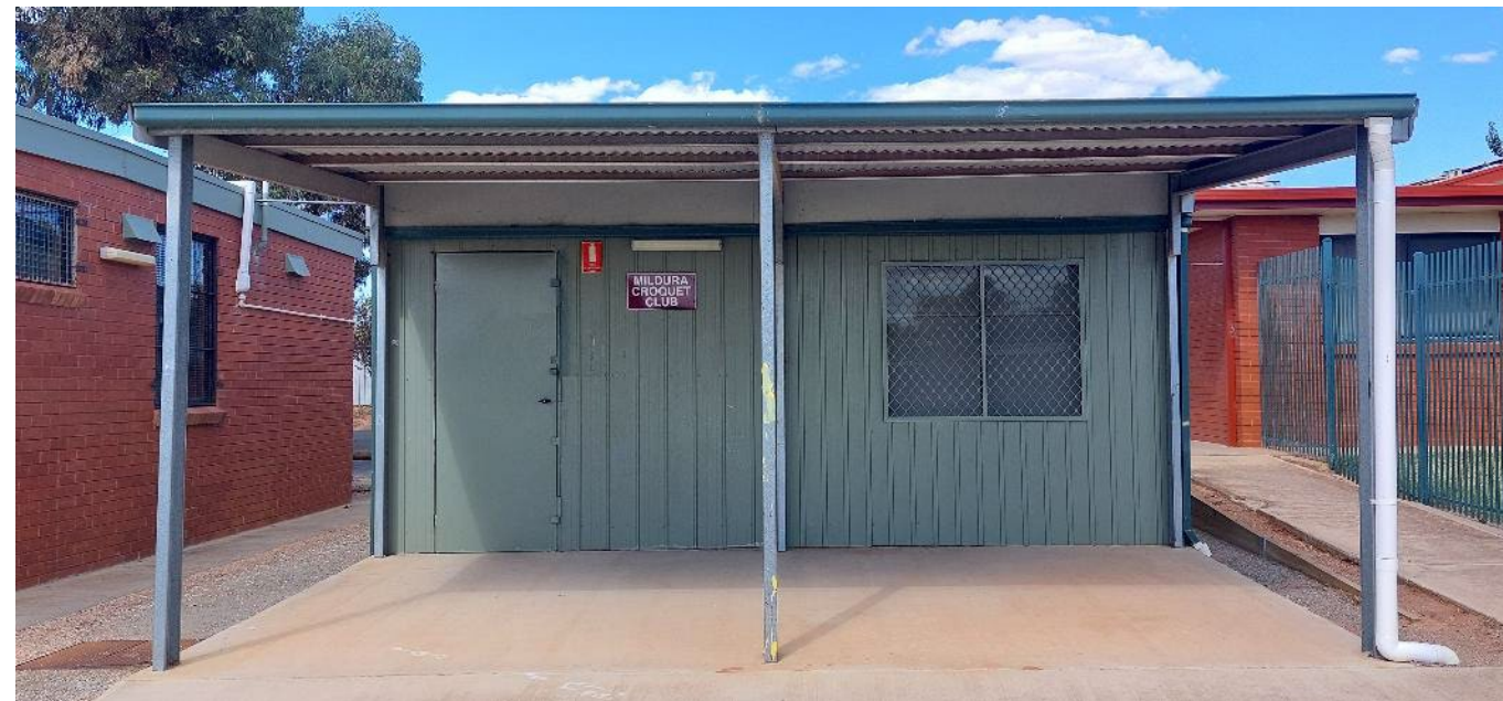
Figure 10 Existing croquet clubroom.
