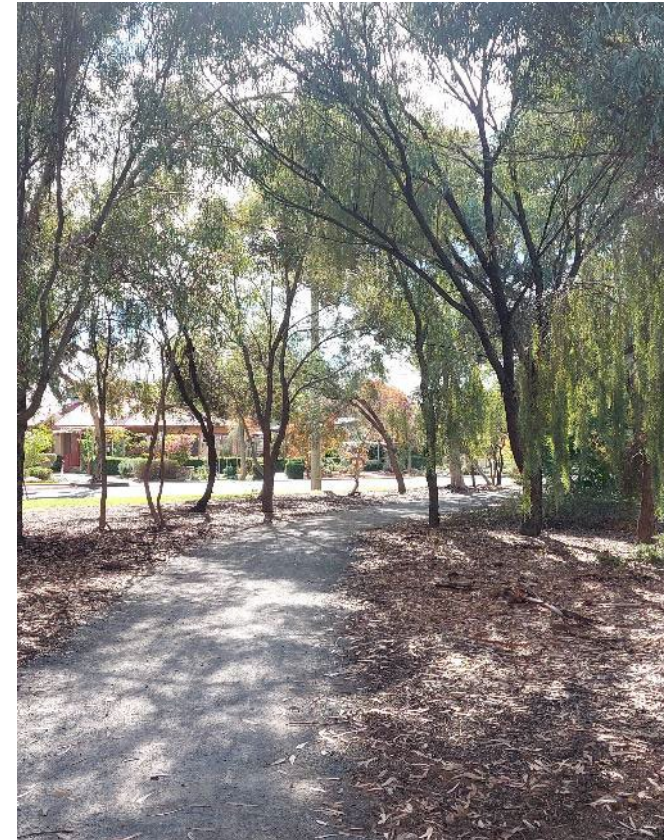
Figure 13 Compacted blue crusher dust gravel boundary path
